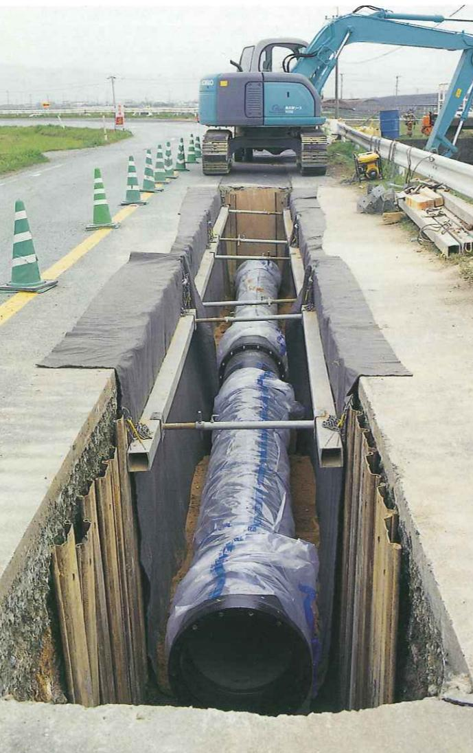
Polyethylene sleeves being used to protect Ductile Iron Pipe.
